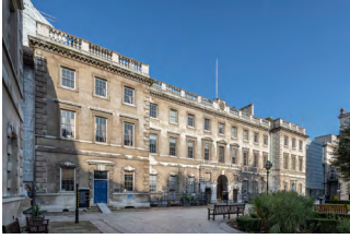
North Wing building
