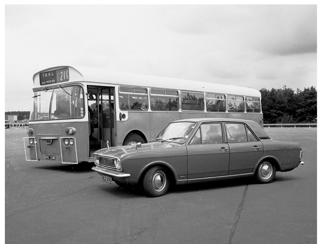
Self driving vehicles at the Transport Research Laboratory in the 1970s - a Daimler bus and Ford Cortina
