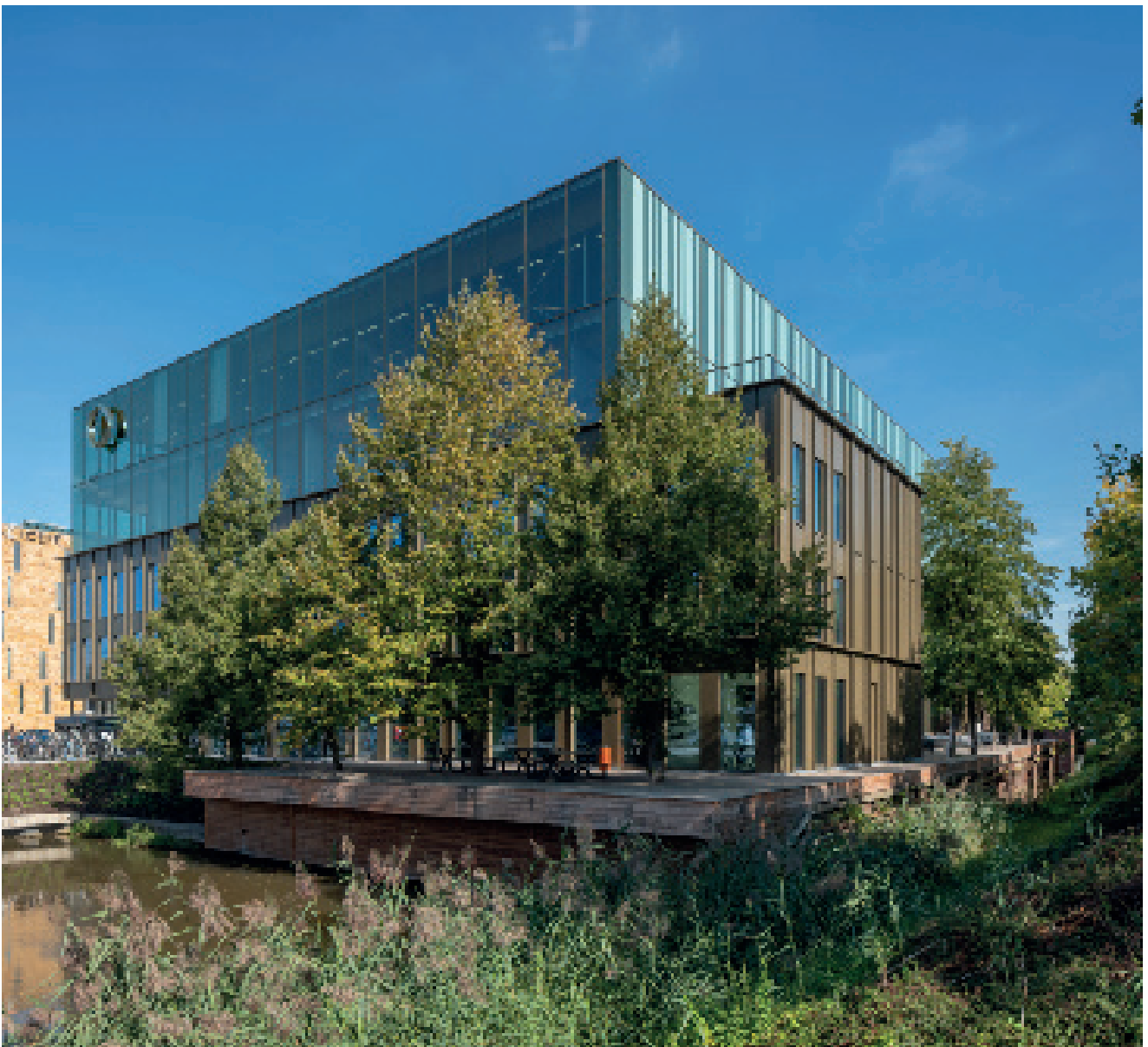
Olympic Edge building, Amsterdam - Credit: Frank Jansen (Edge) photographers Ossip van Duivenbode and Tillemann
