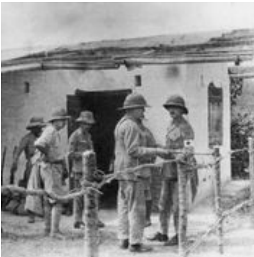
Temporary operating theatre
