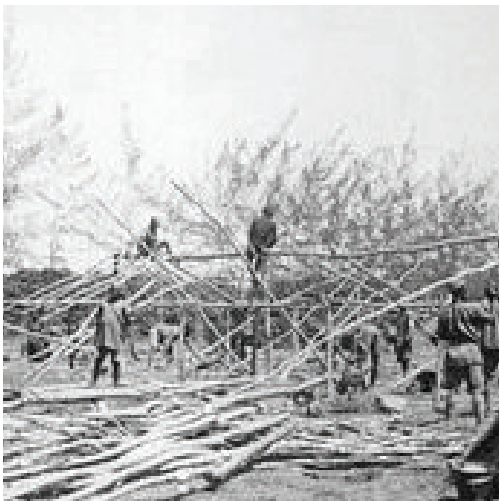
Constructing a banda
